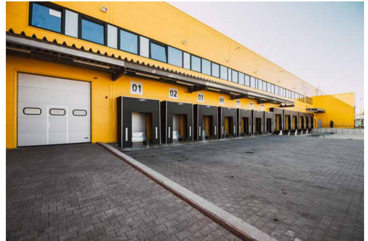
To the south of the hall is the area for delivery and loading of goods from vans and light commercial vehicles. On the south side are located 3 Finger - PuD I (31.66 - 4.14 m), PuD II (31.66 - 4.14 m) and PuD III (22.65 - 4.14 m), with 54 roller shutter doors with sealing sleeves and overload bridges. Fingers have steel support structure. The facades of the hall and PuD I, PuD II and PuD III are lined with NCS S 0580-Y10R composite panels.
